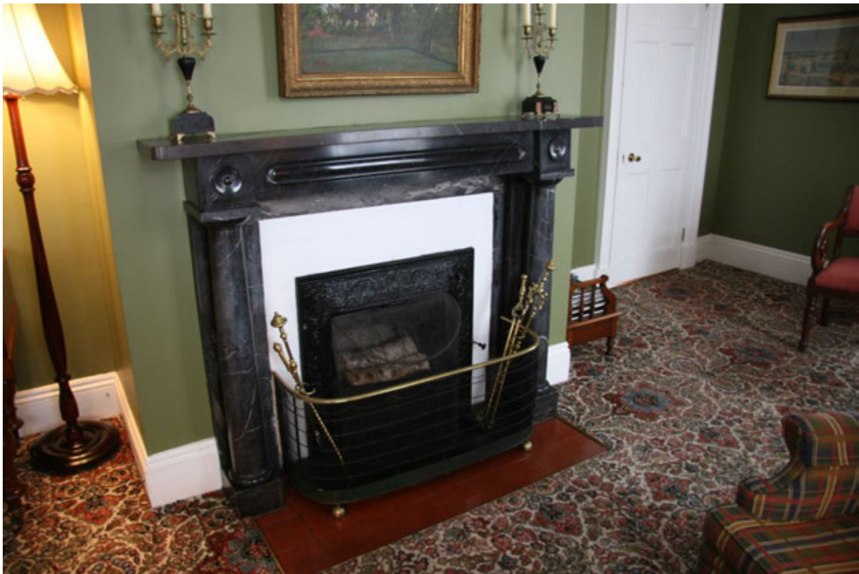
Original marble fireplace in the Governor's Office. At a later time an insert, much like a Franklin stove, was inserted to provide more efficient heating.
