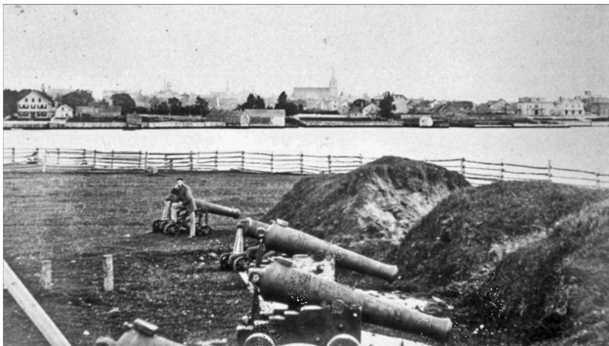
A circa 1860 photo of the Prince Edward Battery at Fanningbank shows the poor condition of the gun platforms and the eroded earth bastions. This neglect was visible for much of the battery's active life. PAPEI.
