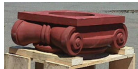
The final full casting in metal of the Ionic capital, based exactly on Smith's original design, but adapted to the larger diameter of the existing columns.
