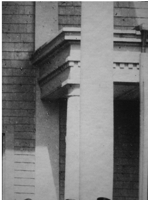
Insertion of veranda entablature into the pilaster of the South portico. Circa 1860 photograph, Porter Collection. It is a neat solution but architecturally perhaps offensive.
