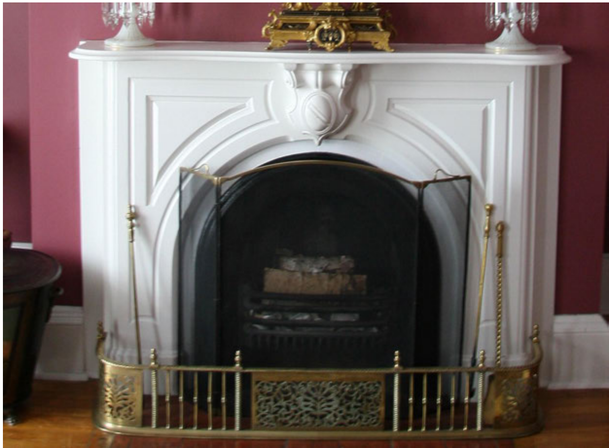
Mass-produced painted slate mantelpiece supplied with coal-burning insert. Circa 1880-90.
